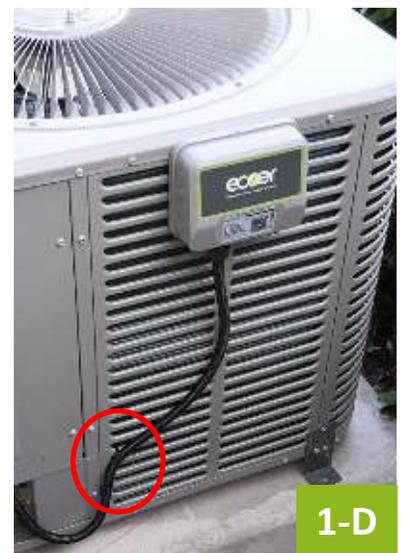
2. Unscrew the cable locker cap and securely fasten the **waterproof joint** to the reserved hole (plug has to be removed).
