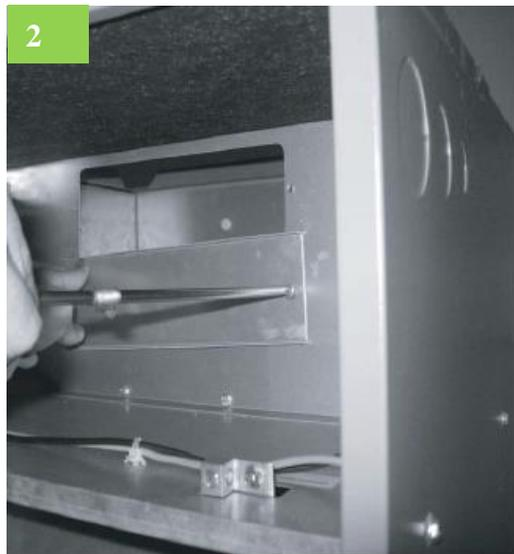
**STEP 3.** Slide the kit into the duct and fasten the element (e.g. attachment and wires).
