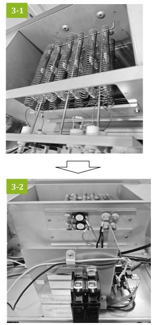
**STEP 4.** Install the circuit breaker into the mounting rail. Knock off the reserved cover for breaker in blower access panel prior to put it back to the unit.
